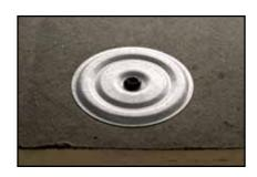
**TOP VIEW**Correctly installed plate/fastener.
