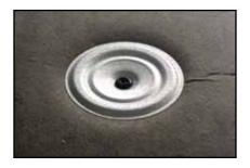
**TOP VIEW**Incorrectly installed, overdriven plate/fastener.
