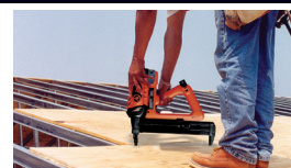
Plywood attachment—using TrakFast plywood to steel pin
